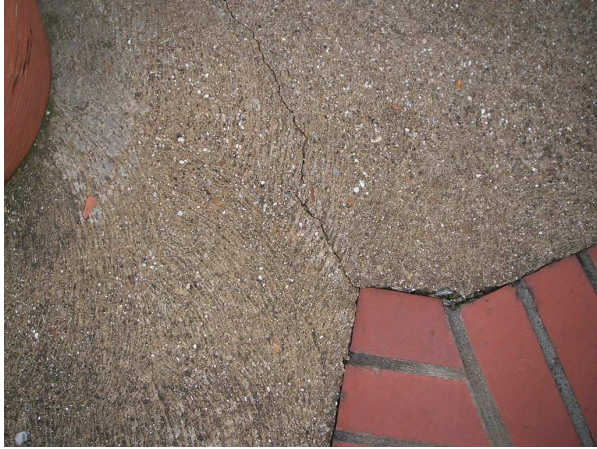
Fig. 12. The crack in the concrete was initiated by a "peak effect" (stress concentration)
