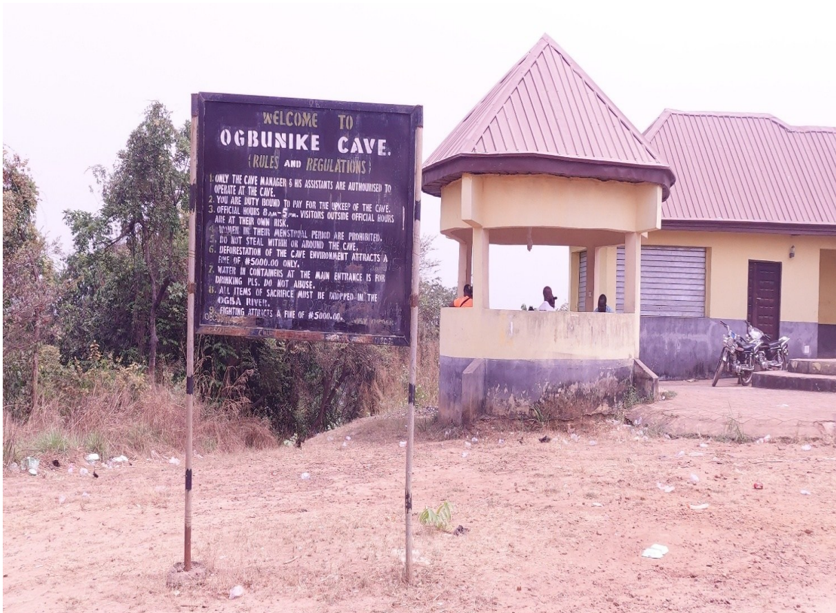
Figure 43: Ogbunike Cave entrance, with visible signpost and access walkway for tourists.
